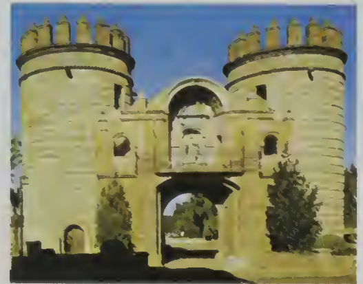
Puerta de las Palmas, ancient entrance gate to city, Badajoz, Spain CIRI—EDISTUDIO
